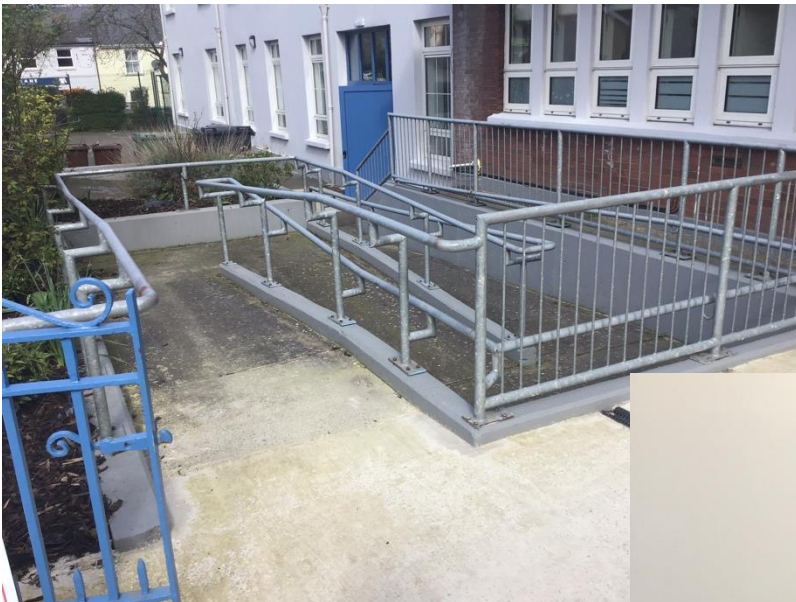
Ramp access to school.
